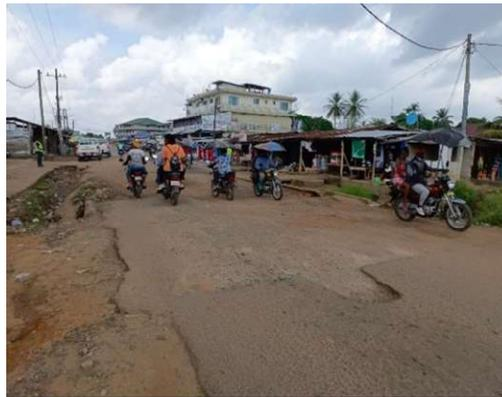
Photos showing critical sections of potholes along Duport Road
