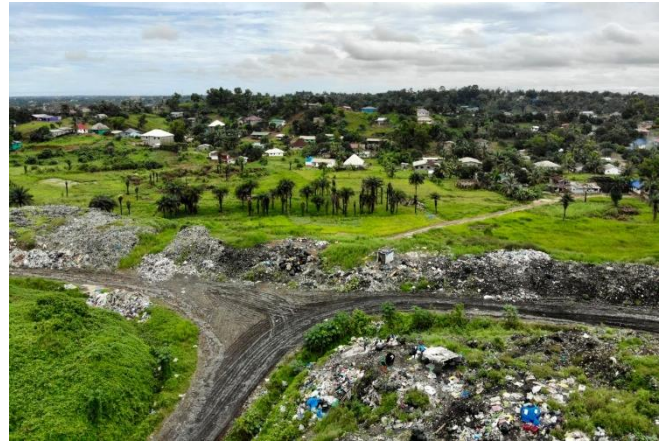
A photo showing an intersection along the access road over the waste leading to the top
