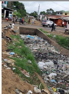
Photo 1: Garbage and siltation in Soniwein Drain (left), Photo 2: Natural drain entering Soniwein Drain near Johnson Street (right)
