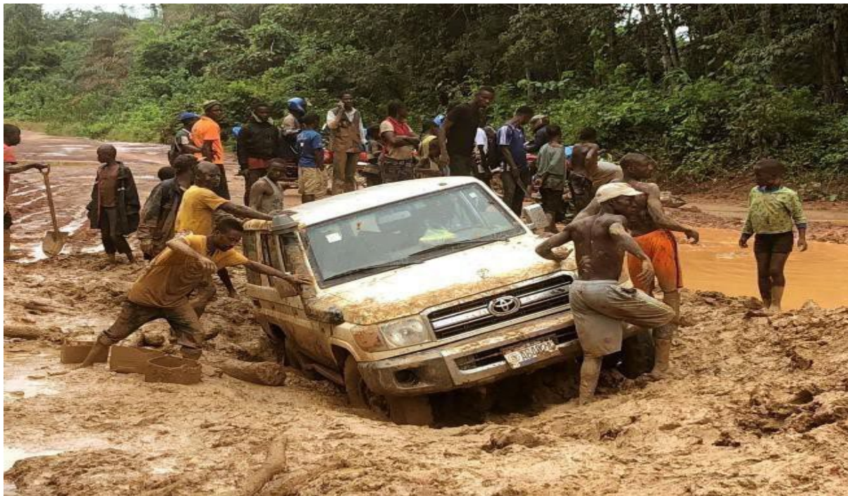
RURAL ECONOMIC TRANSFORMATION PROJECT (RETRAP): TAPPITA TO TOE TOWN (40 KM) ROAD
